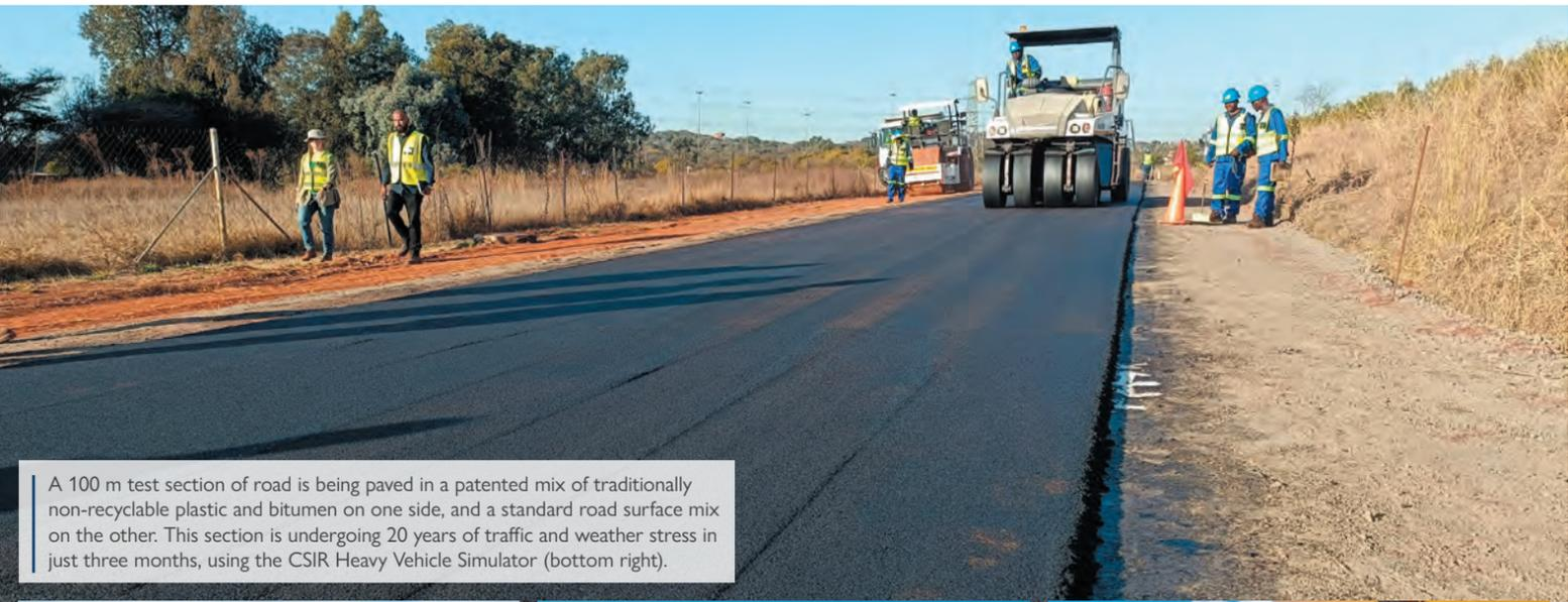
A 100 m test section of road is being paved in a patented mix of traditionally non-recyclable plastic and bitumen on one side, and a standard road surface mix on the other. This section is undergoing 20 years of traffic and weather stress in just three months, using the CSIR Heavy Vehicle Simulator (bottom right).
