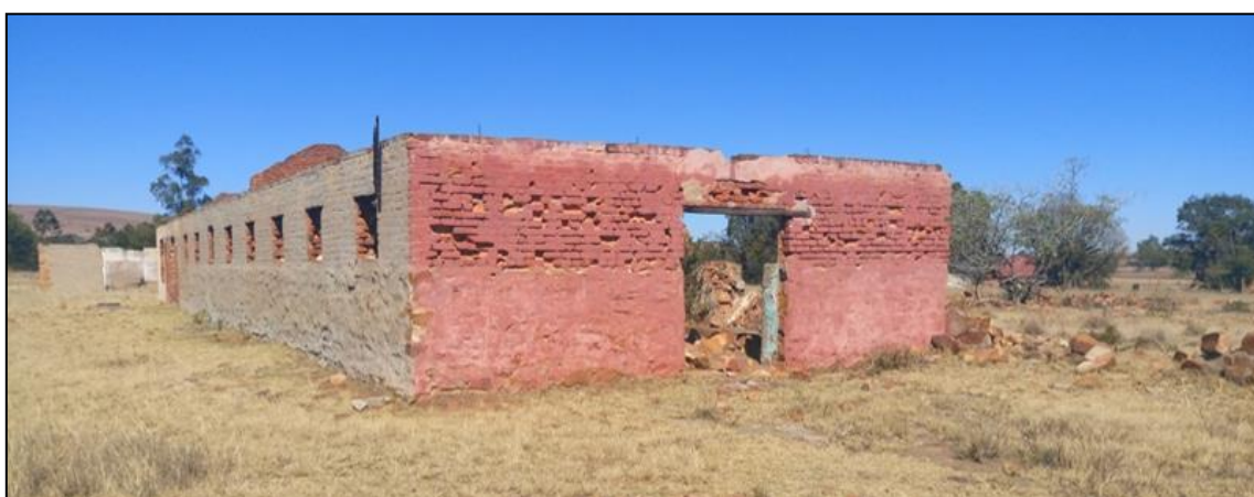
Figure 13: View of the northern wall of the main dairy building showing modern bricks with a concrete lintel above the doorway. The stone and cement kraal is visible to the right.
