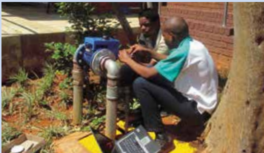
CSIR interns Mla Vilakazi and Matome Montja installing the SmartSense technology to monitor 33 water meters and three pressure sensors on the CSIR campus in Pretoria.
