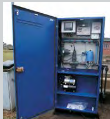
A real-time monitoring system for wastewater.
