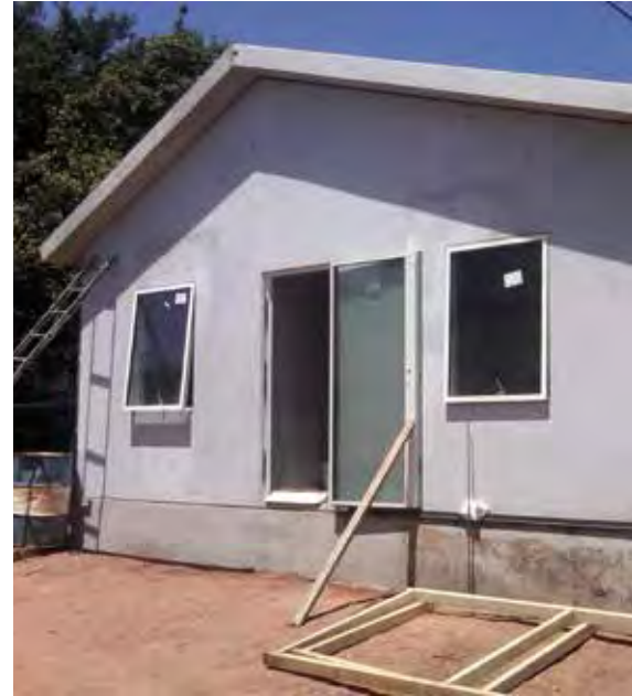
A demonstration house constructed at the CSIR using manufactured housing technologies suitable for South African conditions.
