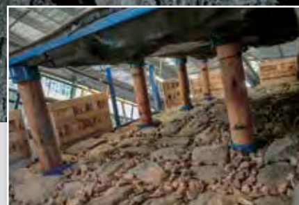
Above and top of page 23: Simulated gold stope with variable dip up to 30 degrees.
