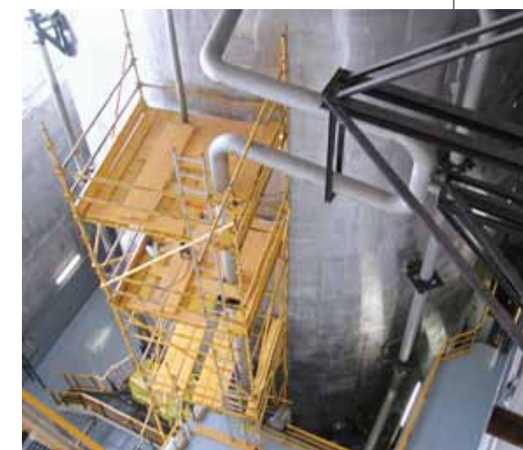
The water storage tank at Koeberg that has been repaired with a new laser process, while in use.
